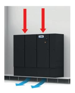
Version for perimetral installation inside the Data Centre with raised floor height less than 550 mm. In this case, the plinth with fixed height of 550 mm is supplied with lateral closure panels and must be installed above the floor. It is essential to check that the height of the ceiling is sufficient to ensure good air suction.
