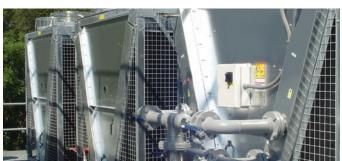
The YVWA chiller can efficiently handle the high condenser pressure required for dry cooling.
