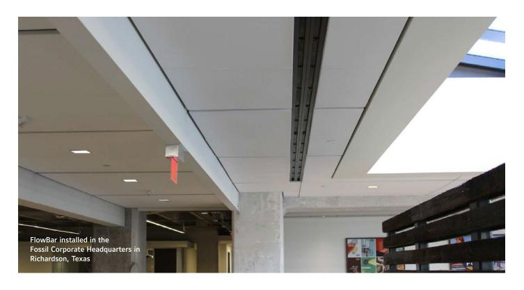
The FlowBar<sup>™</sup> architectural linear diffuser system maximizes maximizes engineering performance without sacrificing aesthetic considerations for the designer. FlowBar's outstanding performance allows higher air flows than conventional linear diffusers, with lower noise levels, making it ideal for high profile designs.
